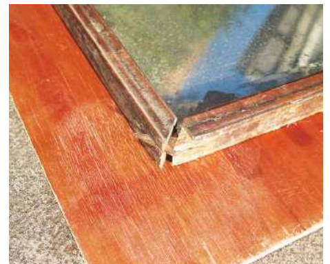
Pic.6 The corner construction
